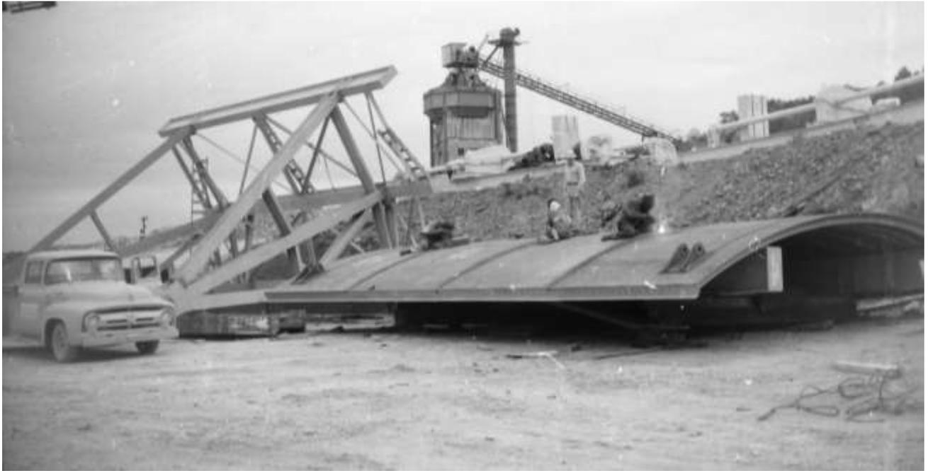
Original field assembly of a Tainter gate at Tulloch.
