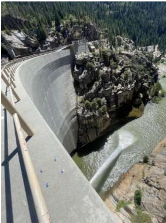
Donnells Vegetation Clearing
