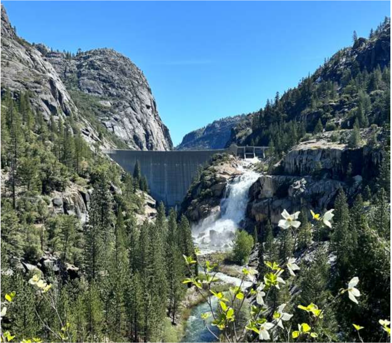
Donnells Dam DSOD Inspection
