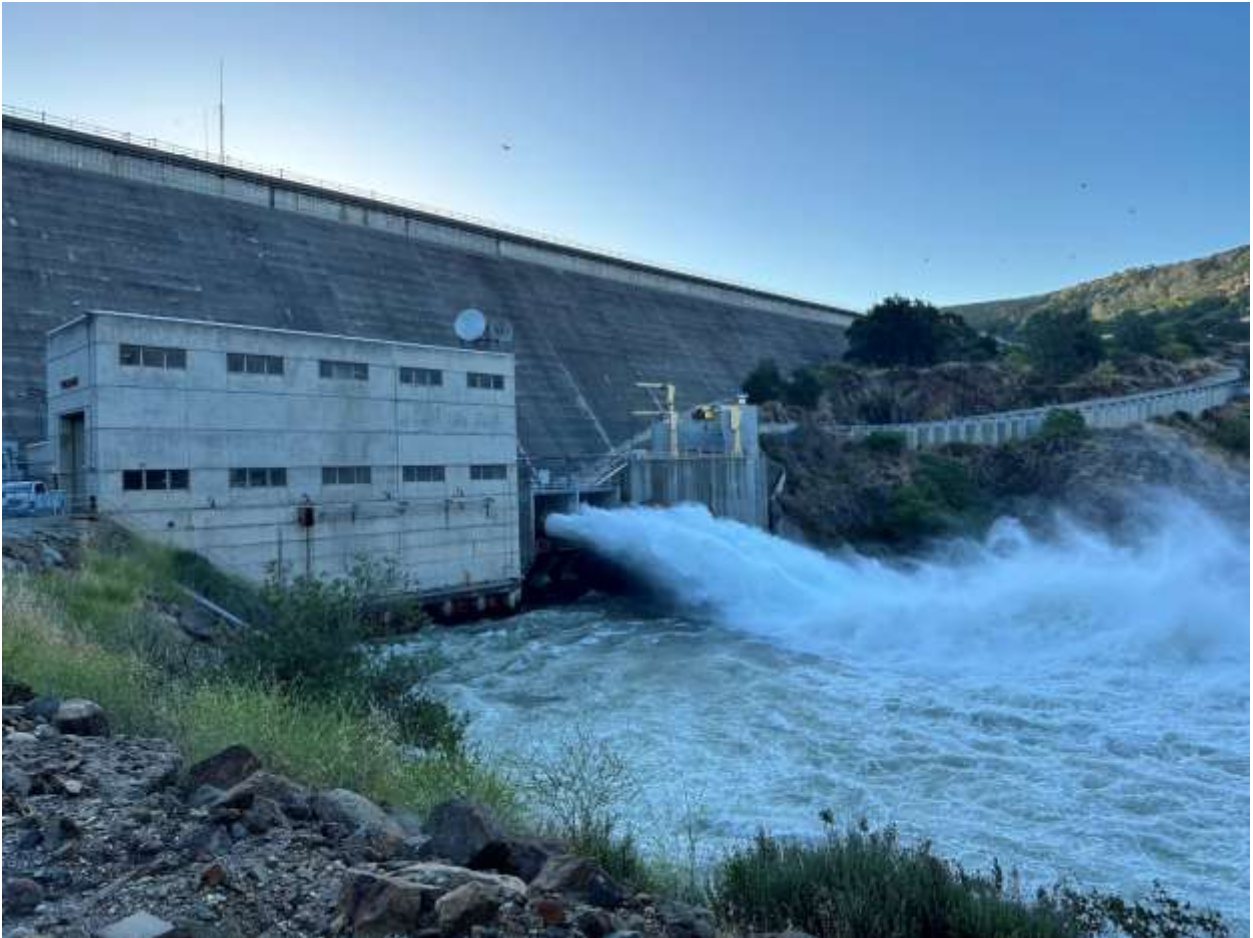
Tulloch Dam and Powerhouse PG&E Outage
