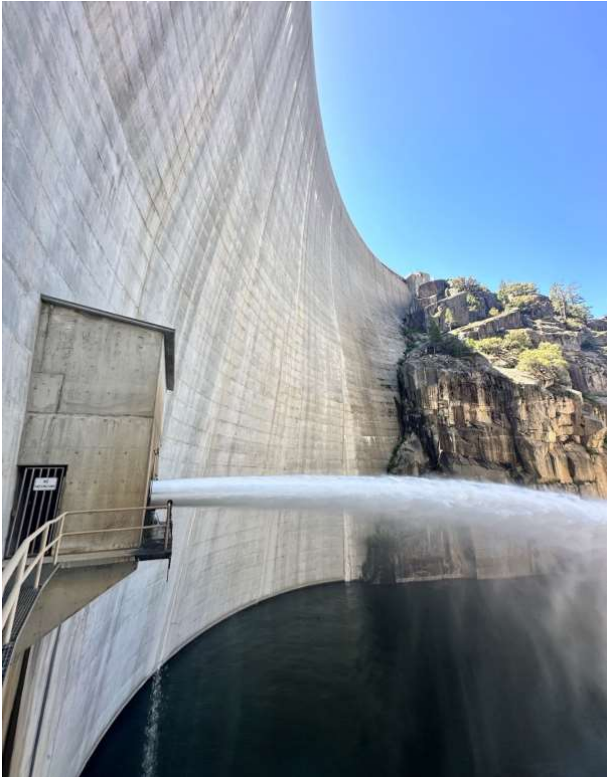
Donnells Dam FERC Inspection
