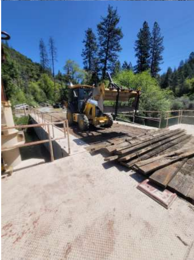
Sandbar Bridge Board Replacement
