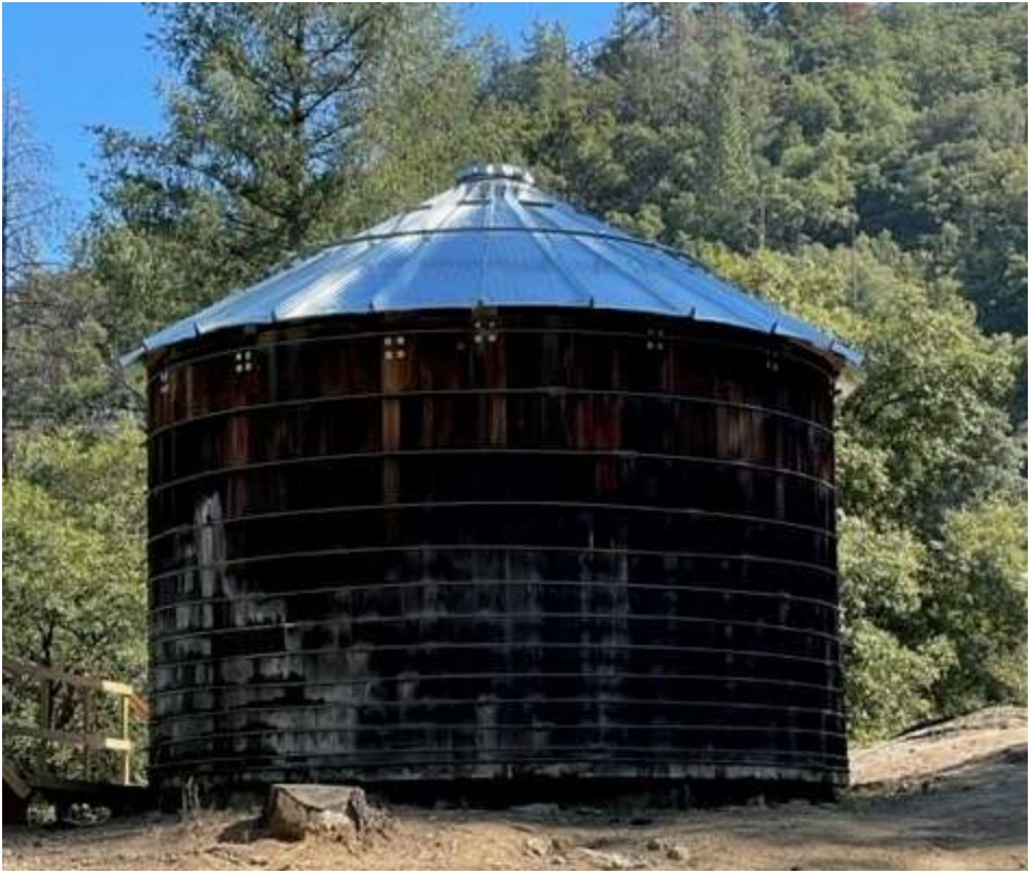
Beardsley Water Tank Roof
