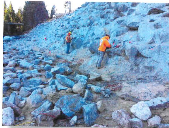
RSP - Eastwood Visitors Center Bank Stabilization
