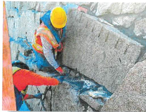
Grouting Stacked Rock - NCPA Union Dam
