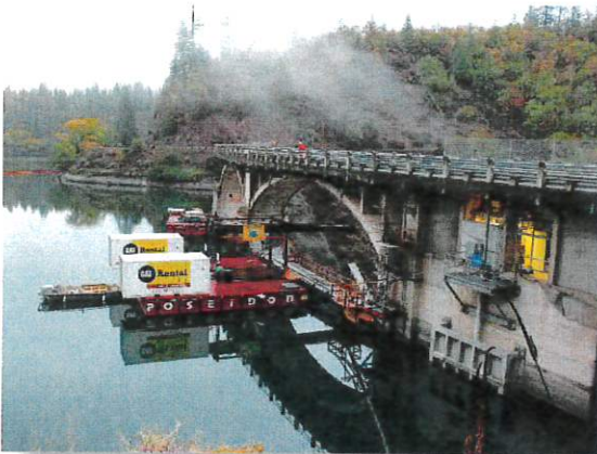
Barge Work – Pit 3 Dam Crest Gate Bladder Replacement
