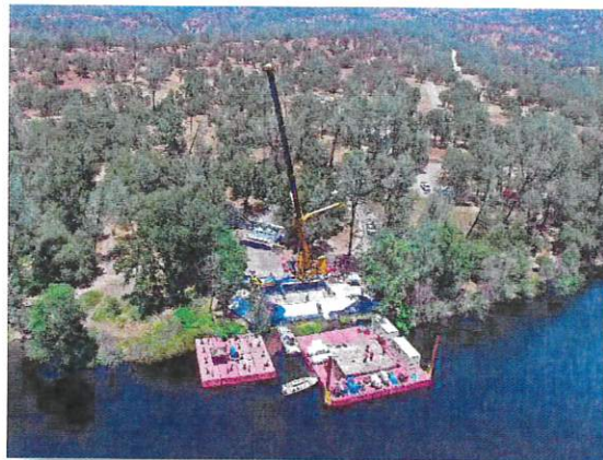
Barge Work – Kerckhoff Dam Low-Level Outlet Gate Replacement
